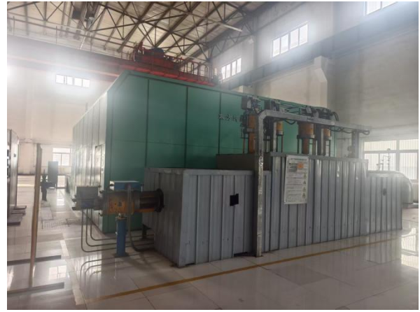
制氧、汽轮发电机隔音罩
