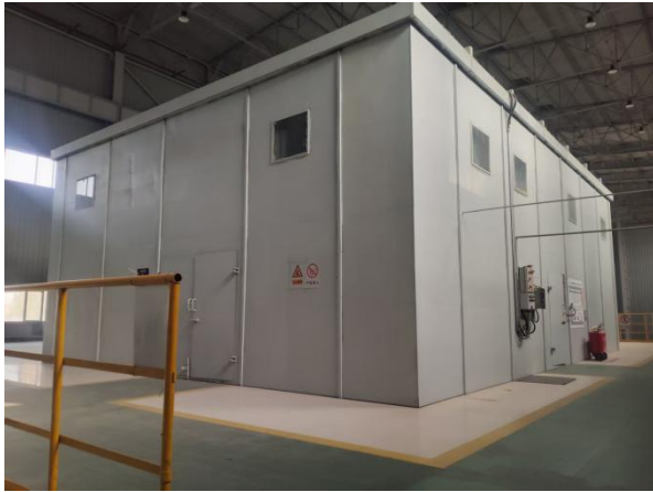
制氧、汽轮发电机隔音罩
